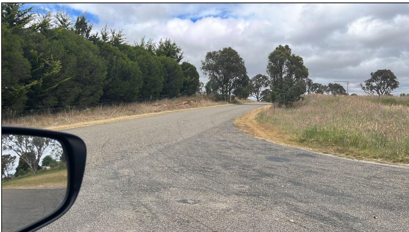
Figure 18: Turton Place and Patemans Lane intersection — view south. Sightlines are about 180 m, with a slight downhill grade towards the intersection from the road's crest. A tree to the right of the road within the reserve reduces sightlines.
