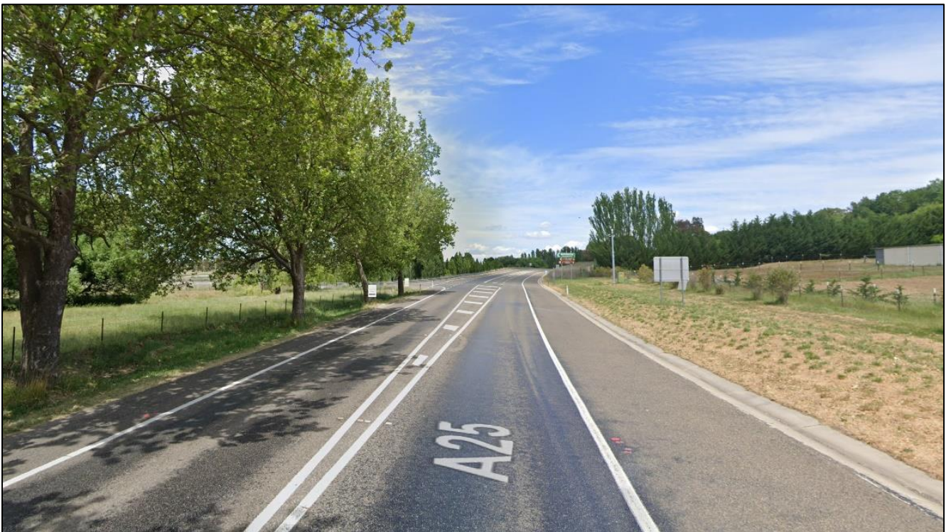
Figure 4: Barton Highway, looking south towards the intersection with Murrumbateman Road (Source: Google)
