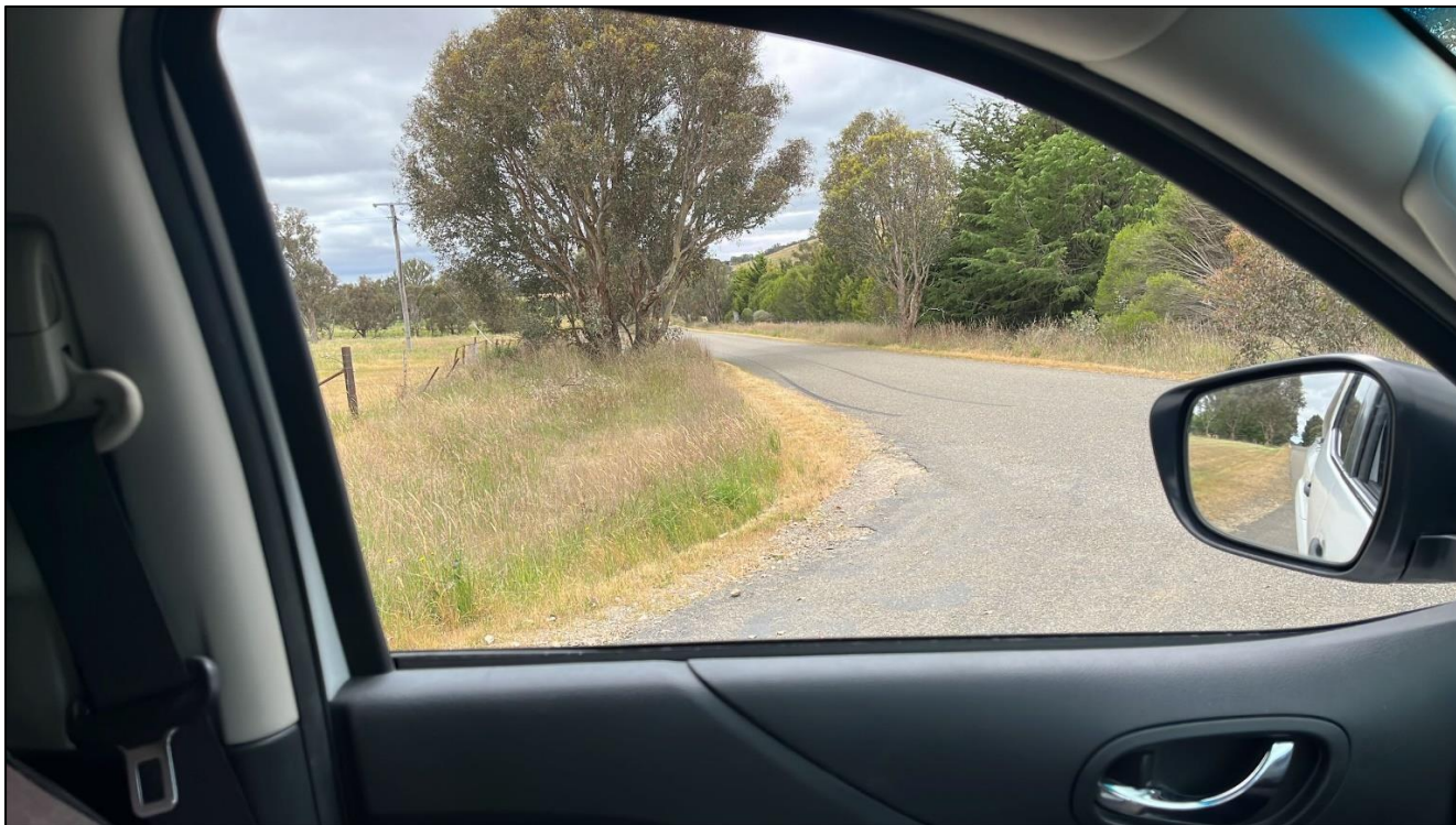
Figure 17: Turton Place and Patemans Lane intersection – view north, the sightlines are restricted to 120 m due to a tree in the road reserve
