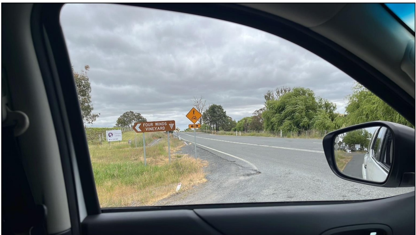
Figure 15: Patemans Lane at the Murrumbateman Road intersection – view northwest (about 200 m)
