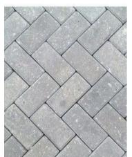
2.12. Paver - General Maintenance Washing down the pavers with a hose or a high pressure domestic cleaner is not recommended until the pavers have settled and the grout sand has set between the paving joints. The best type of sand to use between the joints is a dried sand or a polymeric sand best known as Pave Set or similar
