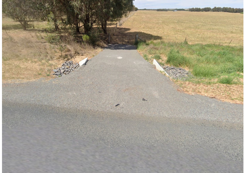
Figure 2.9: Existing Access to Proposed Lot 1 (Source: Google Maps Street View, January 2025)
