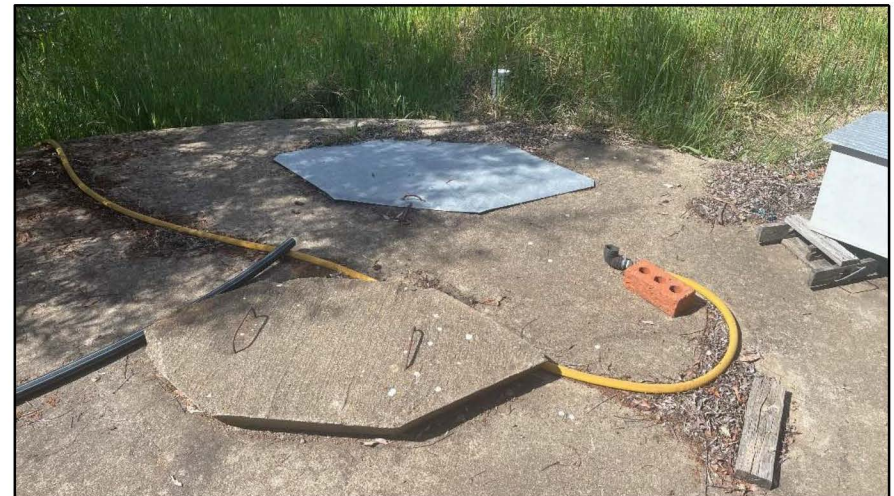
Figure 27 – Large underground concrete water tank with hatches. (McGregor, 2024)
