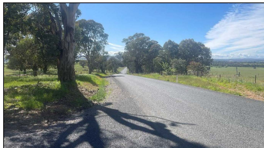
Figure 10 – Looking east on Back Creek Road towards Sutton Road. (McGregor, 2024)
