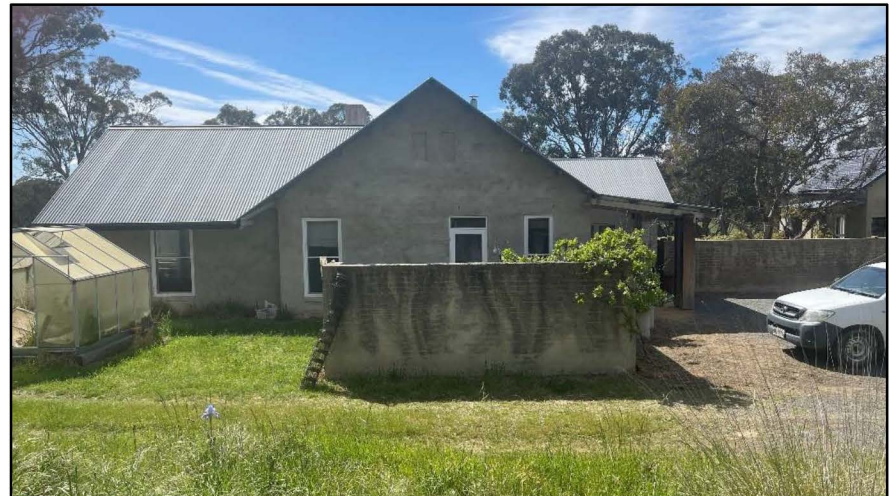
Figure 26 –Western façade of the existing dwelling. (McGregor, 2024)
