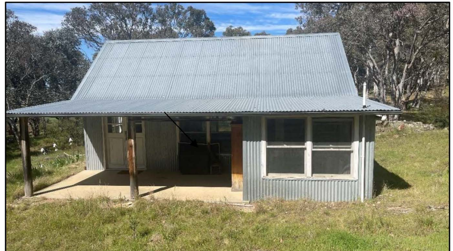
Figure 26a –Storage shed near the two concrete water tanks. (McGregor, 2024)
