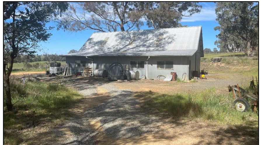
Figure 27a – Existing farm shed with access road. (McGregor, 2024)
