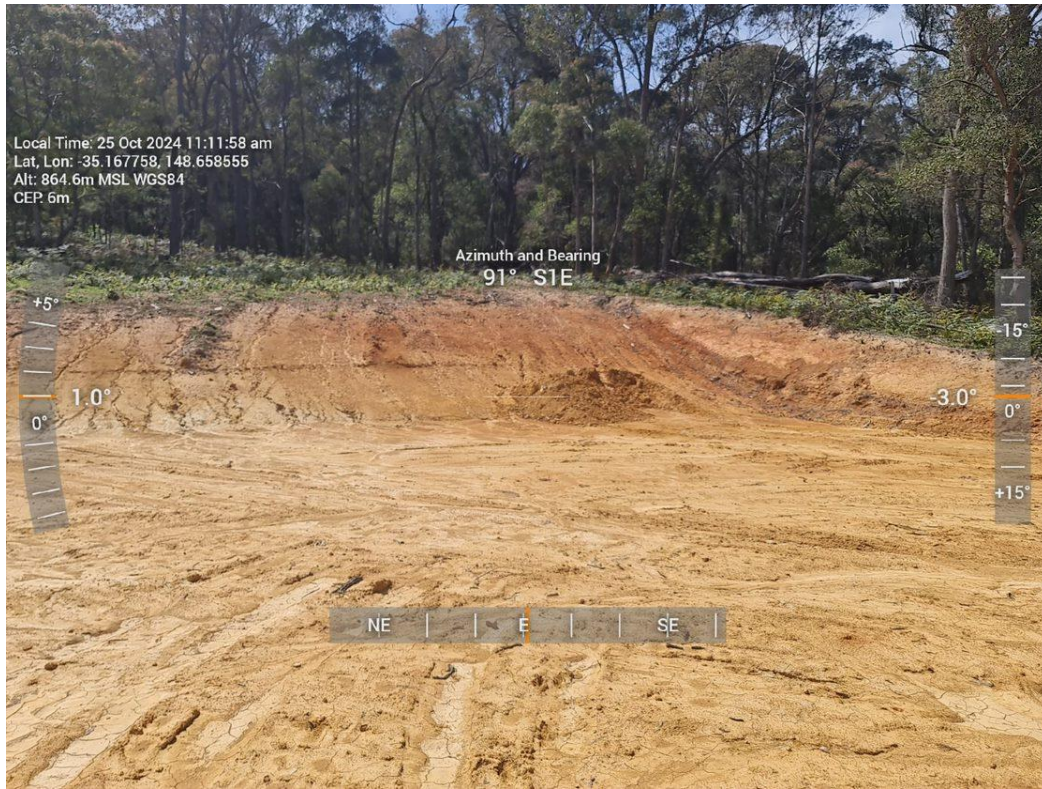
Figure 9: Looking east across Lot 2.
