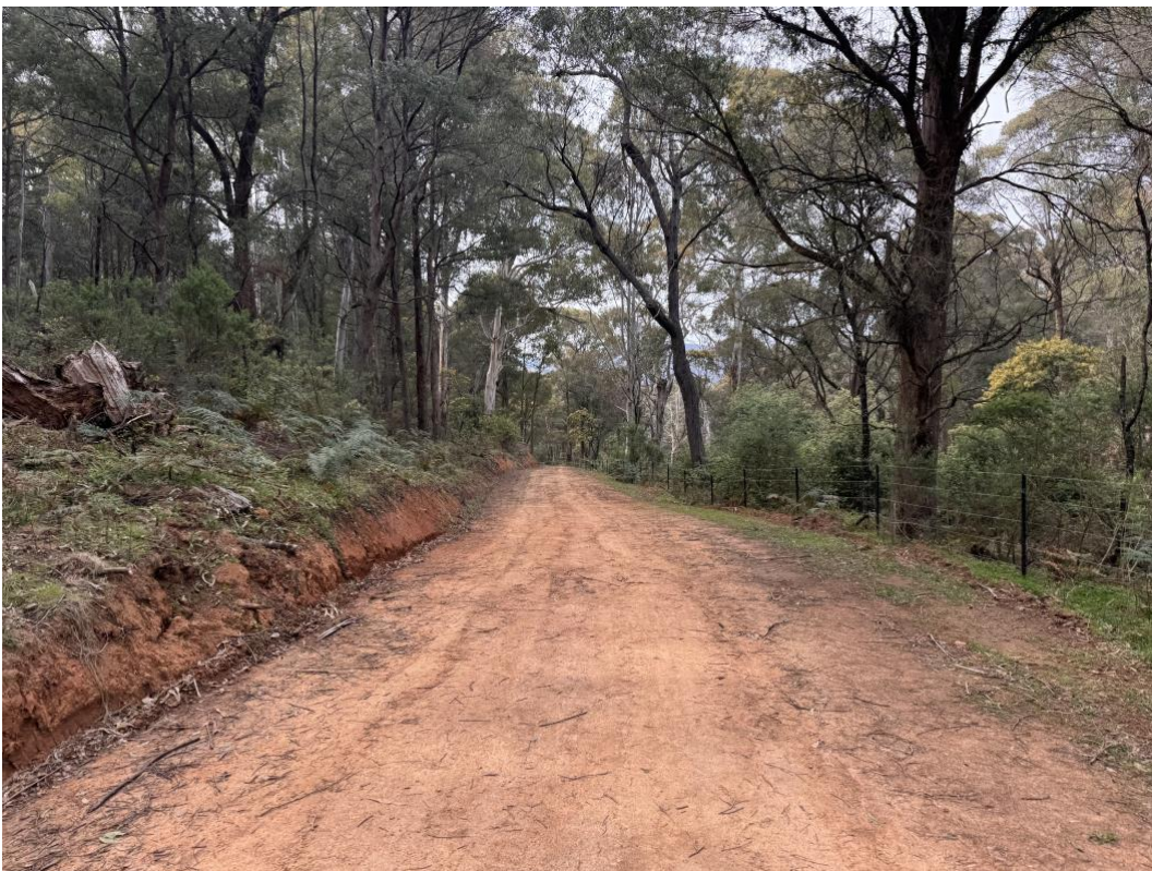
Photo 6, Example of existing internal tracks & fencing in very good condition.
