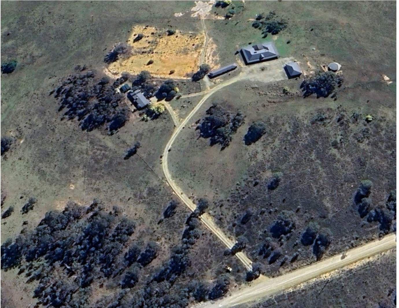
Figure 2.14: Existing Access Track on Proposed Lot 1 (Source: Google Earth Aerial Imagery, October 2024)
