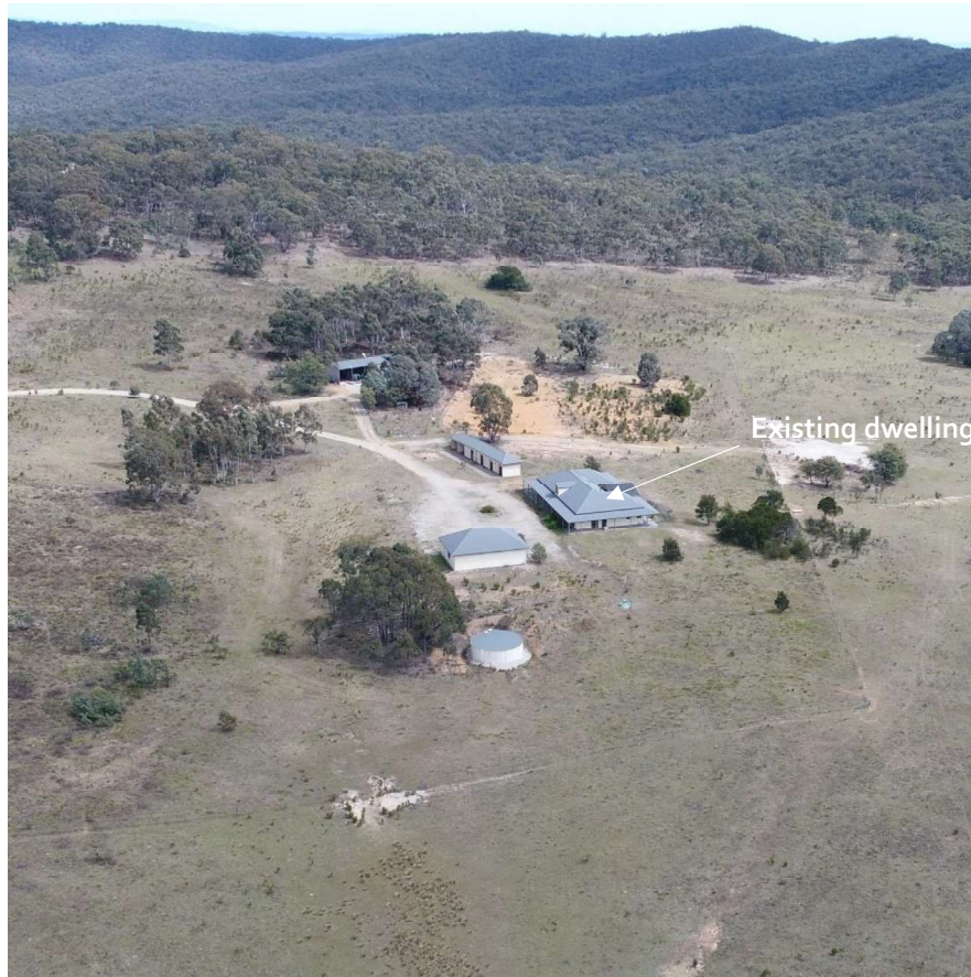
Figure 23 – Existing dwelling and three Class 10a structures. (McGregor, 2024)
