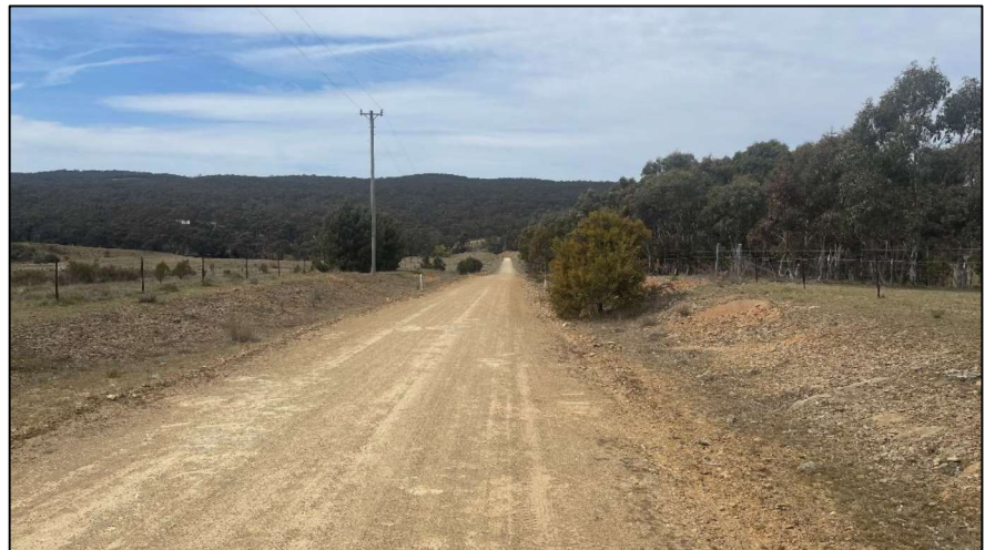
Figure 10 – Well-formed public no through Beralston Road. (McGregor, 2024)
