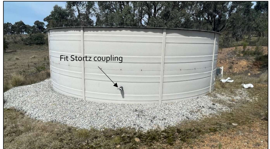
Figure 26 – Existing 90,000L metal water tank, Stortz coupling required. (McGregor, 2024)
