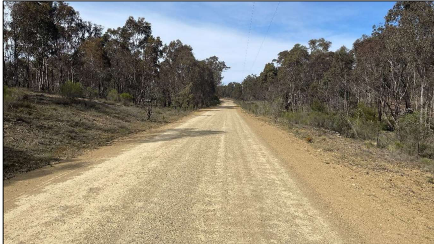
Figure 7a – Looking south on Beralston Road. (McGregor, 2024)
