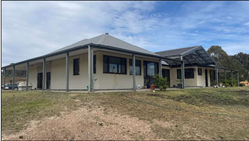
Figure 24 – Northwest and northeast facade of the existing dwelling. (McGregor, 2024)
