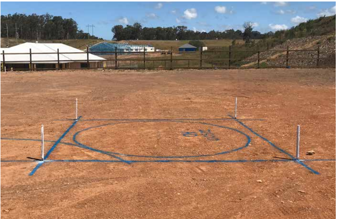
Rainwater Tank Ground Mark out
