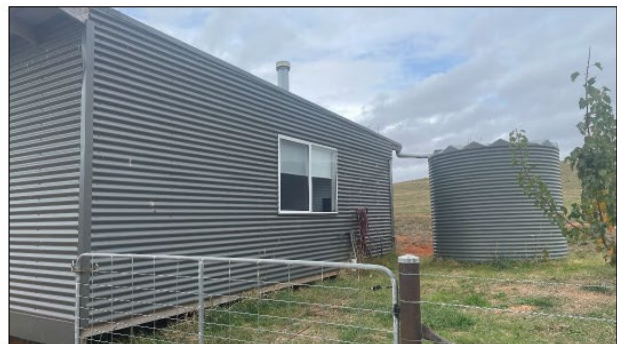
Figure 93 – If possible fit a Storz coupling to the outlet of the existing water tank
