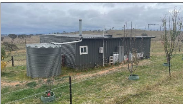
Figure 92 –South facia of the existing dwelling. (McGregor, 2024)
