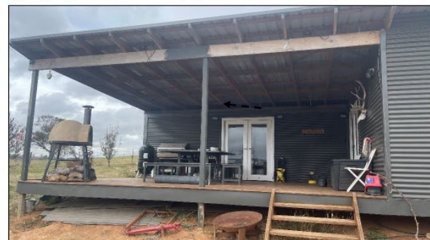
Figure 94 – North facia of the existing dwelling. (McGregor, 2024)
