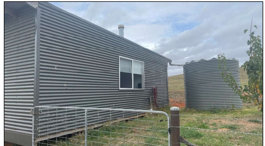
Figure 93 – If possible fit a Stortz coupling to the outlet of the existing water tank
