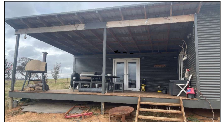
Figure 94 – North facia of the existing dwelling. (McGregor, 2024)
