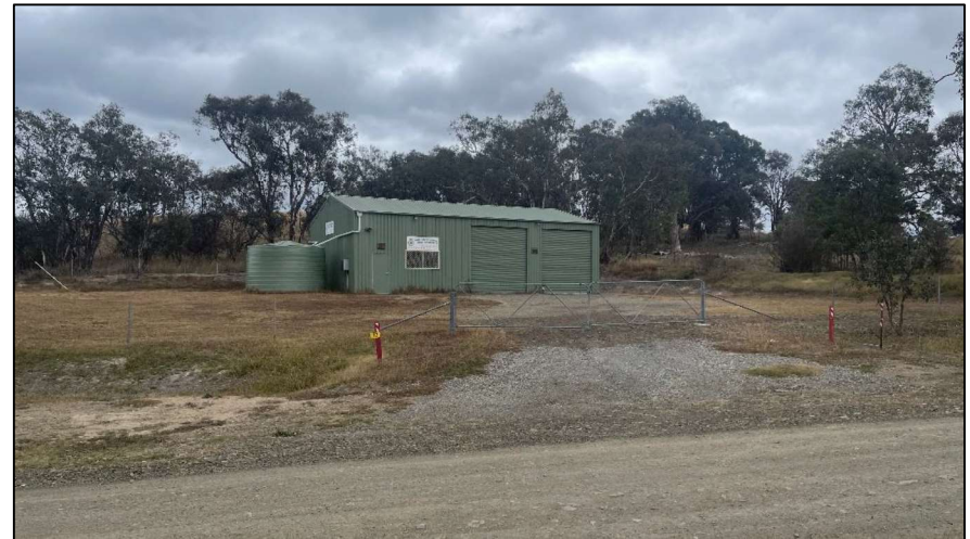
Figure 98 – RFS fire shed opposite Lot 1 entry (McGregor, 2024)
