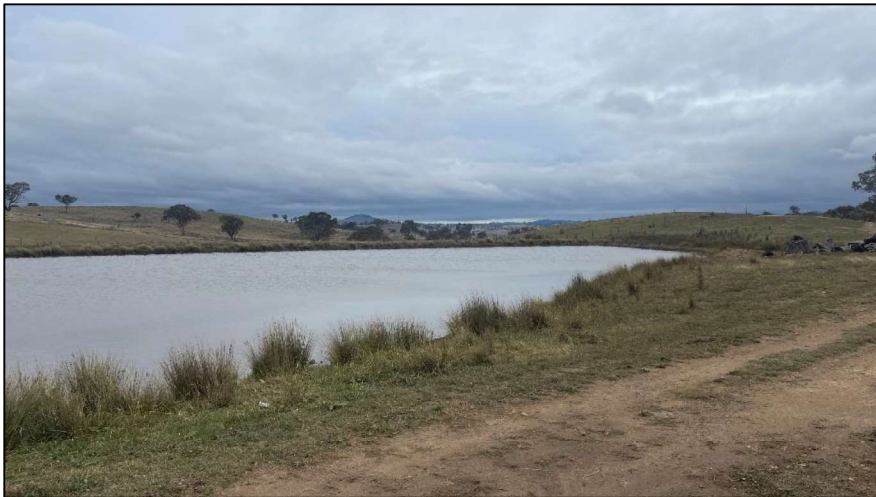
Figure 96 – One of the large dams beside the PAR as a static water supply. (McGregor, 2024)
