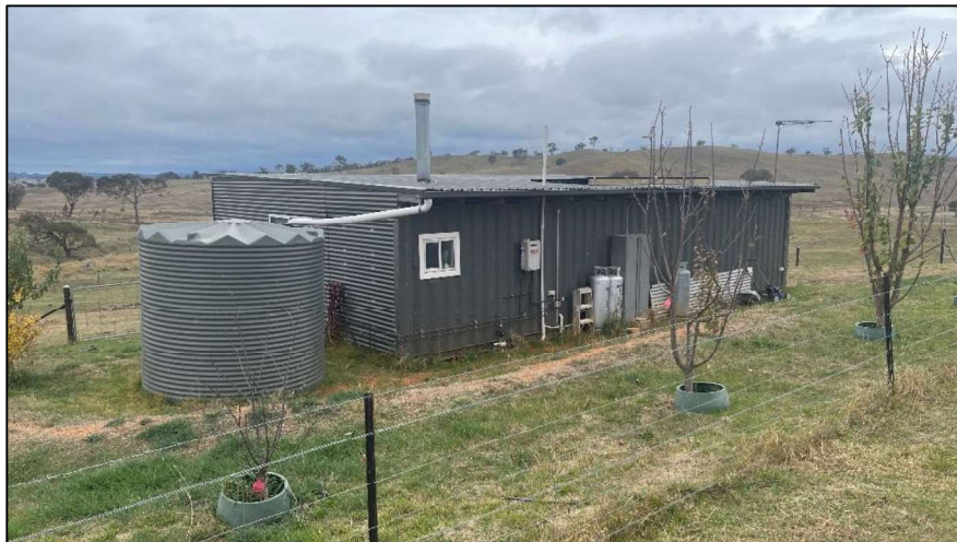
Figure 92 –South facia of the existing dwelling. (McGregor, 2024)
