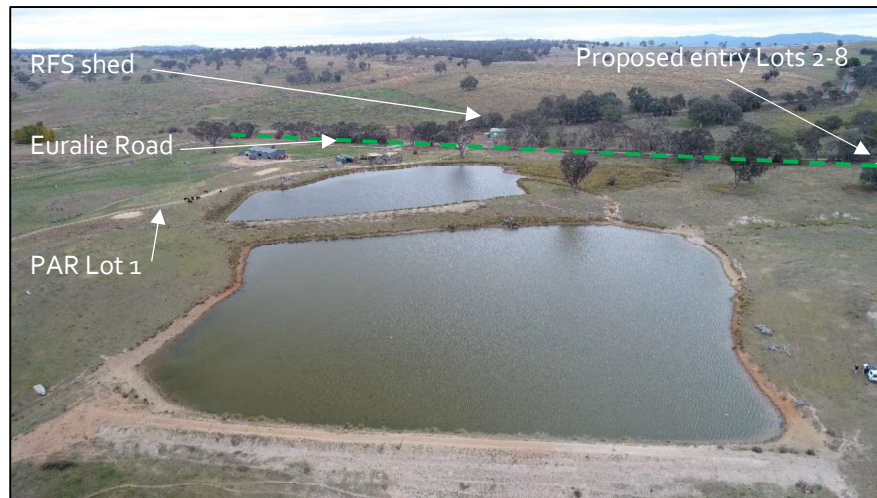
Figure 7 – Looking south showing the two large dams. (McGregor, 2024)
