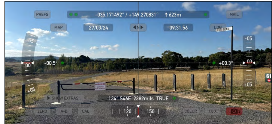
Figure 15. Photo point 7 Looking at the emergency access road at the end of Harcourt Close.
