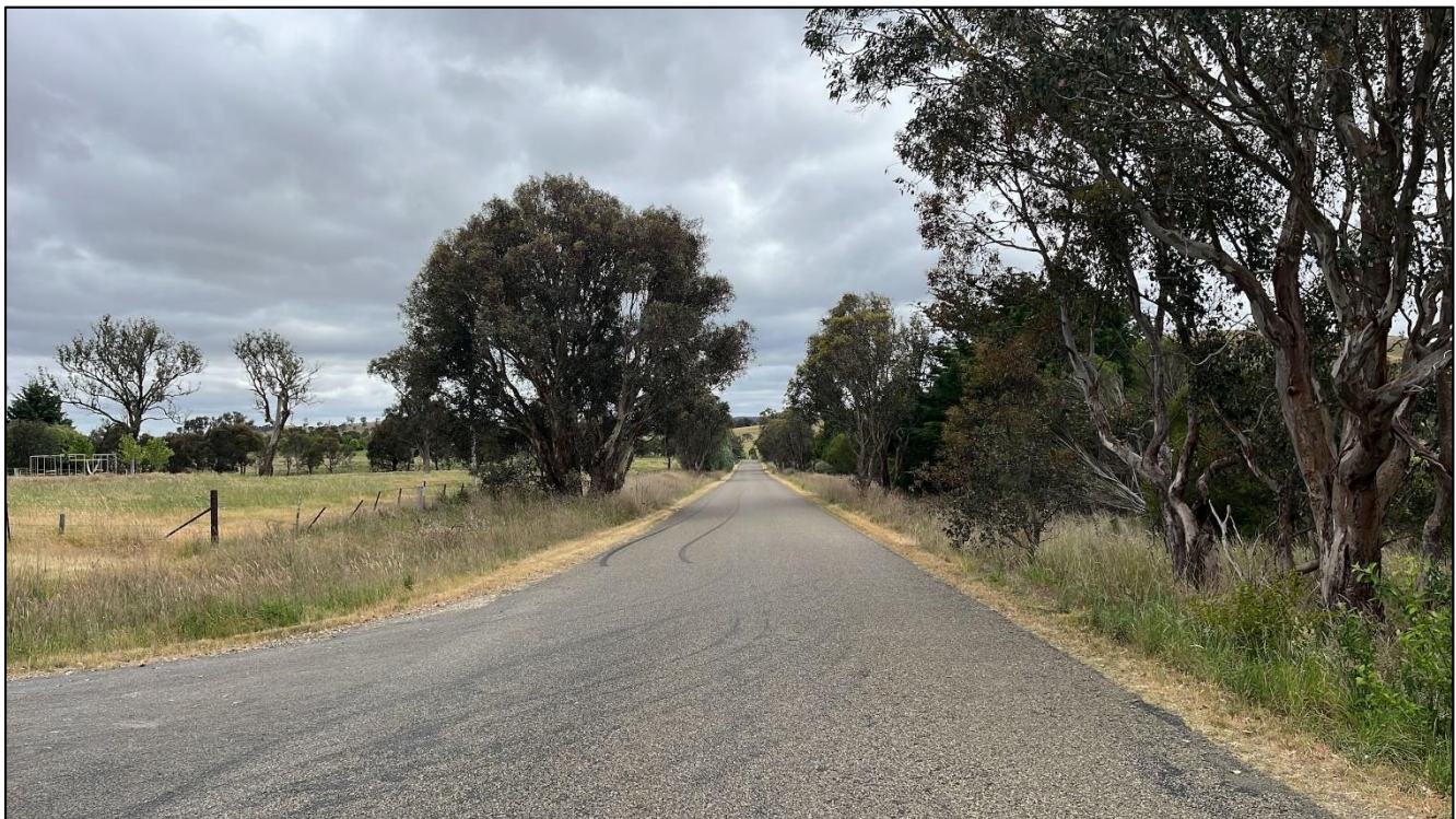
Figure 7: Patemans Lane, looking north from the intersection with Turton Place
