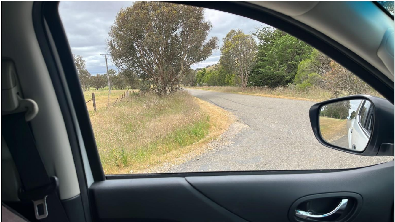
Figure 17: Turton Place and Patemans Lane intersection – view north, the sightlines are restricted to 120 m due to a tree in the road reserve
