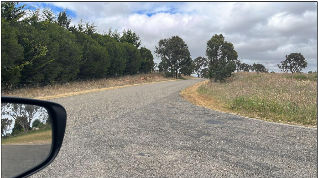
Figure 18: Turton Place and Patemans Lane intersection — view south. Sightlines are about 180 m, with a slight downhill grade towards the intersection from the road's crest. A tree to the right of the road within the reserve reduces sightlines.
