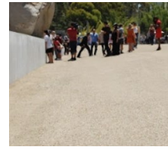
Stabilised decomposed path
